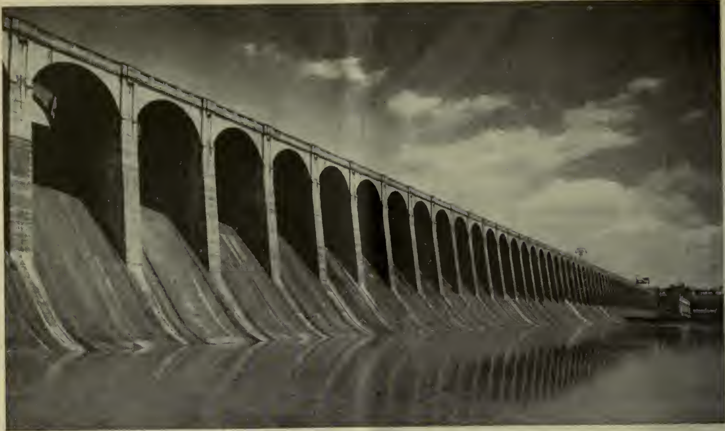
Wilson Dam at Muscle Shoals, Ala., built for use in World War I but incomplete at the Armistice—now part of the TVA system
